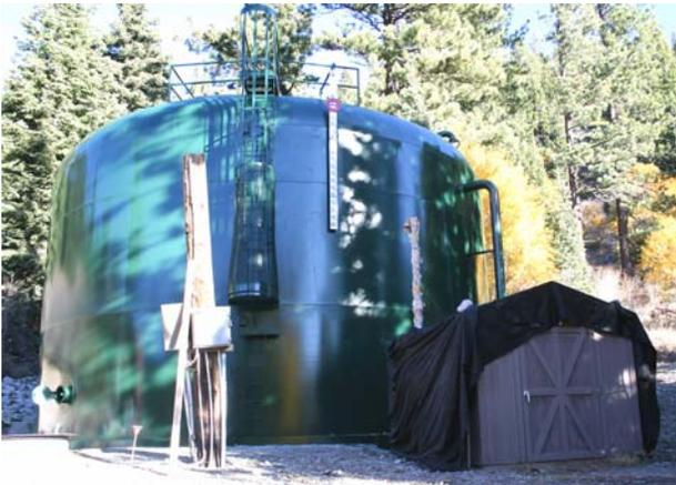
New 160,000 gallon welded steel tank
